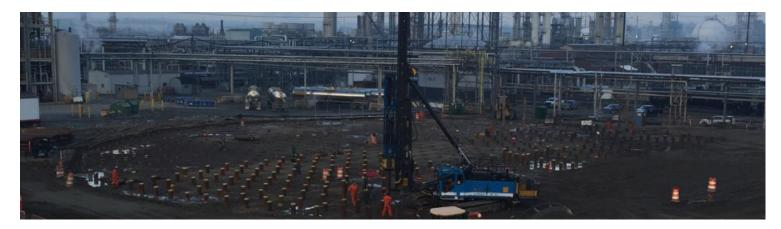
**Consolidated Pipe and Supply** provided over 1,500 pcs. 12.750"OD x .375wall ASTM A252 Grade 3 steel pipe piles for the 900-million-gallon natural gas tank foundation of Sunoco Logistics SXL Mariner East 2 project in Marcus Hook, Pennsylvania. Simpson and Brown, Inc. of Cranford, New Jersey was the pile driving contractor.
